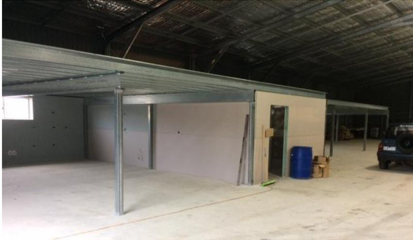
This photo shows the joists in place for the mezzanine floor. A large area where job storage will be ORGANISED !
